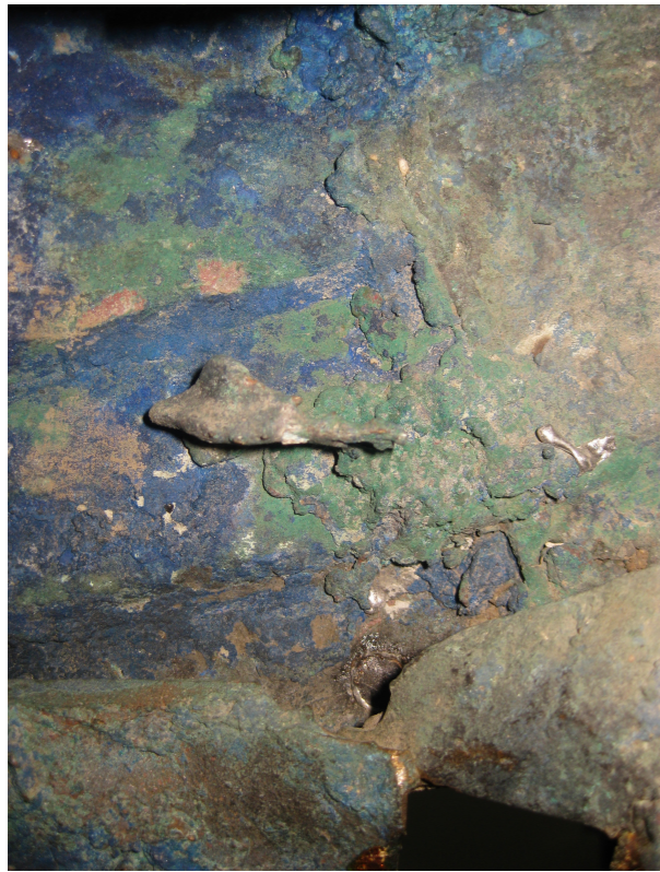
FIGURE 4.15. Apollo: detail, endoscope photo to show interior corrosion
