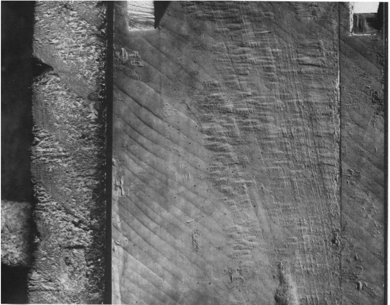
Fig. 3 Examination of an edge reveals concentric growth rings and a tongue and groove joint.
