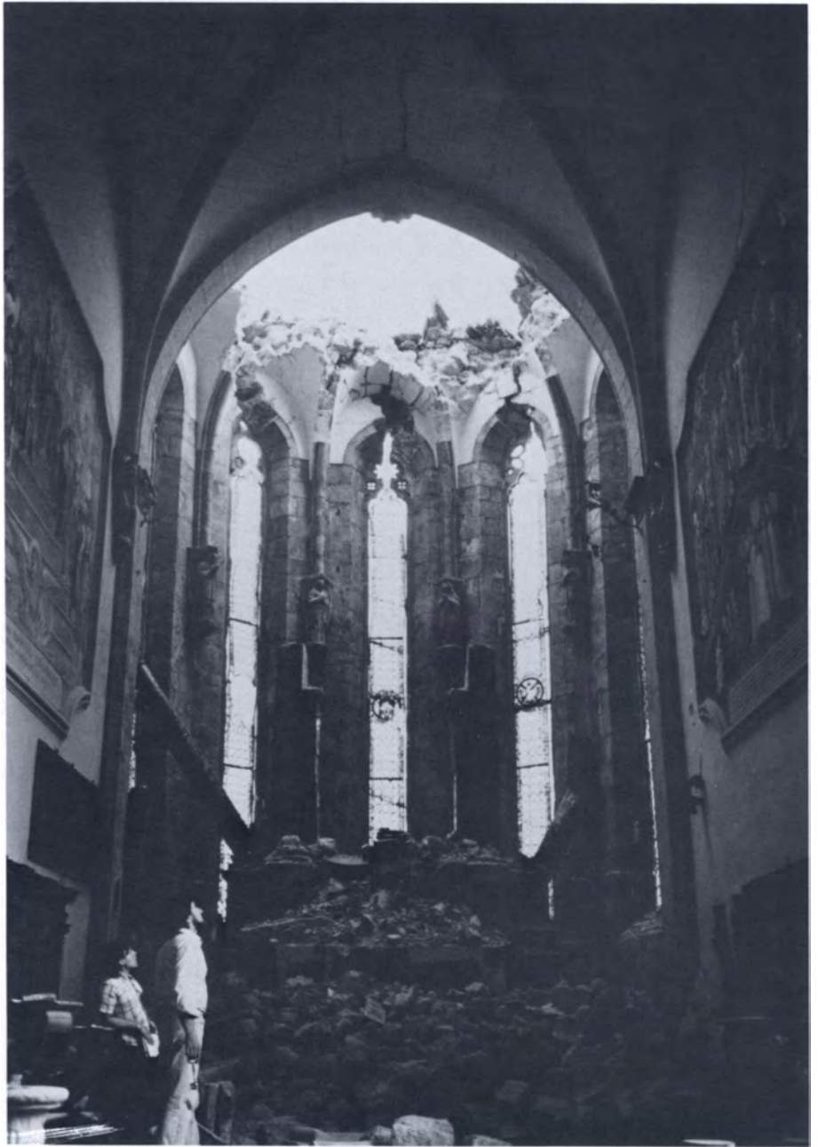
Figure 2. Cathedral after the May 6, 1976 earthquake; Venzone, Friuli.
