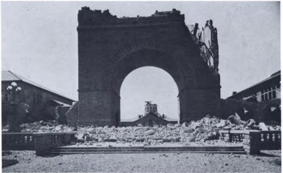
Figure 1. Above: Memorial Arch, Stanford University, California, after the 1906 earthquake. Below: Opposite view of arch. Rather than restore the arch, the top portion was later removed, leaving only two guard towers.
