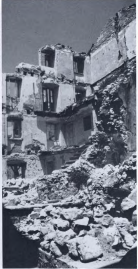
Figure 6. On the other side of the wall, only the shell of the building remains.
