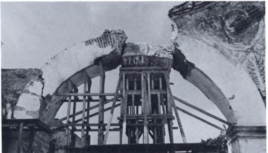
Figure 16 The Arch of San Francisco in Antigua, Guatemala, undergoes restoration efforts following the February 4, 1976, earthquake.
