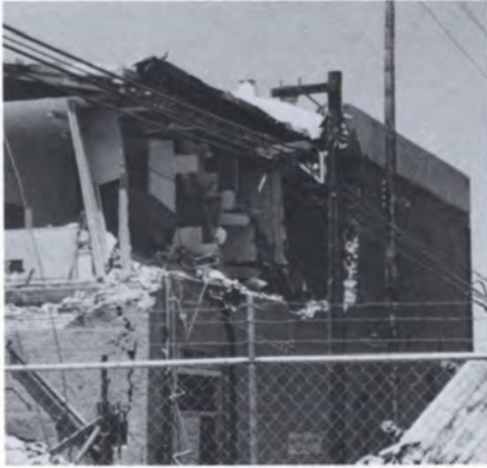
Figure 15 Above: unanchored portion of building collapses in 1983 Coalinga earthquake. Opposite: anchoring of floor joists stabilizes wall.
