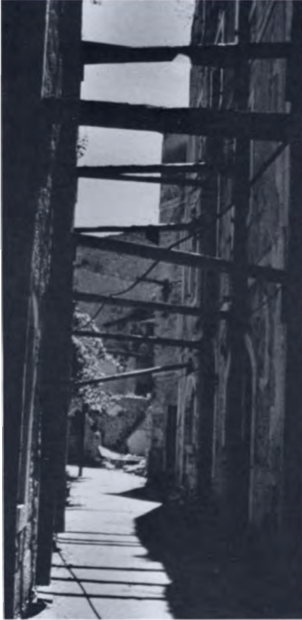
Figure 5. Temporary shoring between two vernacular buildings following 1979 earthquake, Budva, Yugoslavia.
