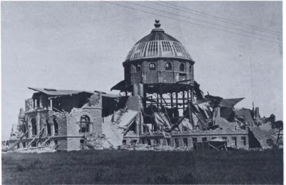
Figure 17 Above: Stanford University's domed library shortly before the 1906 earthquake, Palo Alto, California. Below: Damage was so extensive, the building was later completely demolished and never rebuilt.
