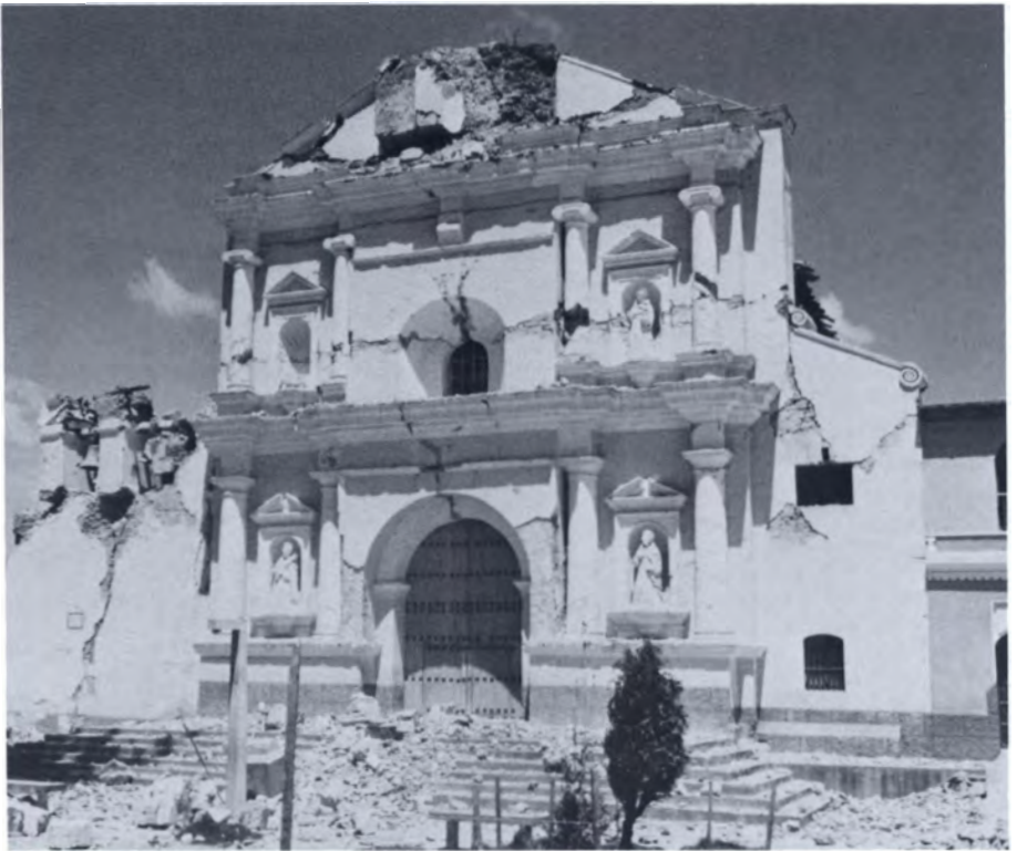
Figure 3. Cathedral with cracking above arches caused by February 4, 1976, earthquake; Tecpan, Guatemala.
