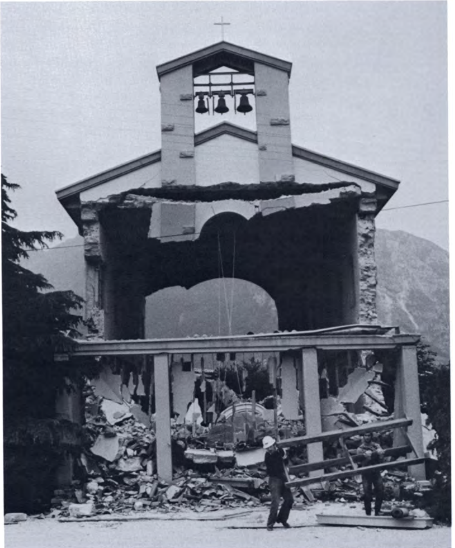
Figure 11. Surviving roof and bell tower following the 1976 earthquake, Gemona, Italy.
