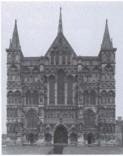
Figure 2. Salisbury Cathedral, west front. Photograph courtesy of the Courtauld Institute of Art.
