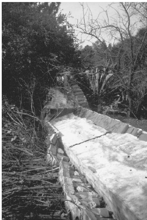
Figure 5.7 Mid-height, out-of-plane flexure damage.
