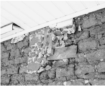
Figure 7.15 Numerous repairs to wall at tie-rod end plate (De la Ossa Adobe, Encino, Calif.).
