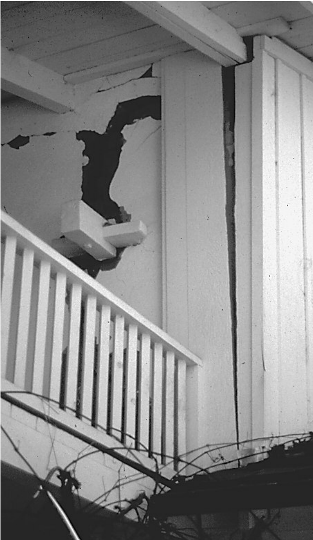
Figure 7.17 Damage to wall adjacent to wood anchor (Rancho San Andres Castro, Watsonville, Calif.).
