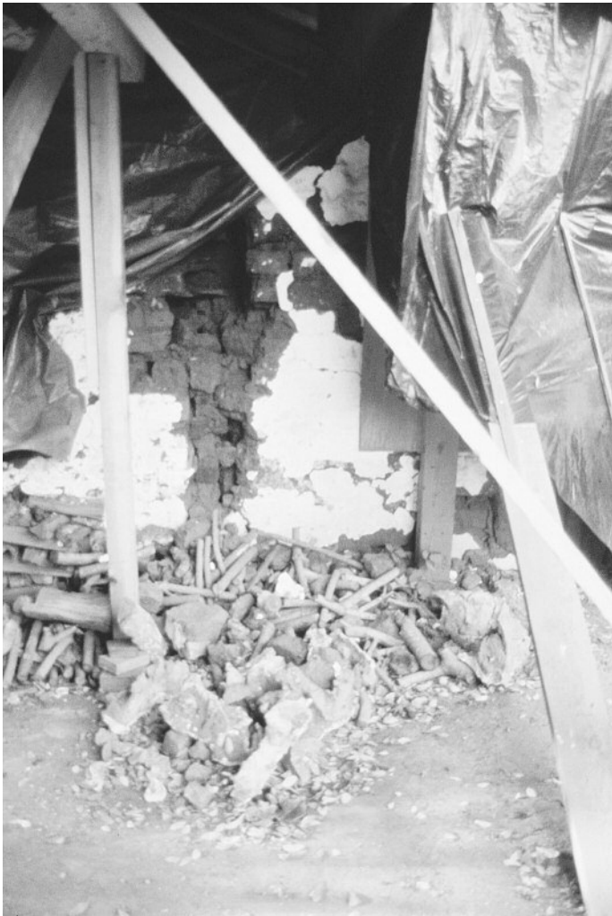
Figure 1.8 Rancho San Andres Castro Adobe, Watsonville, Calif., showing failure of early concrete repairs to adobe after the 1989 Loma Prieta earthquake.
