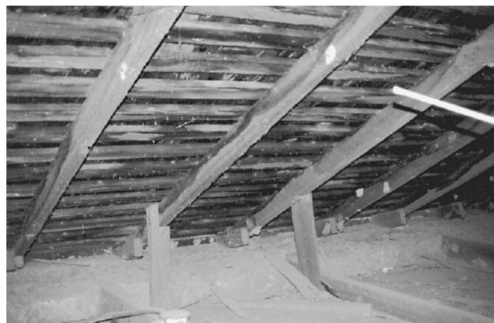
Figure 7.9 Roof framing resting on, but not attached to, the top course of adobe bricks.
