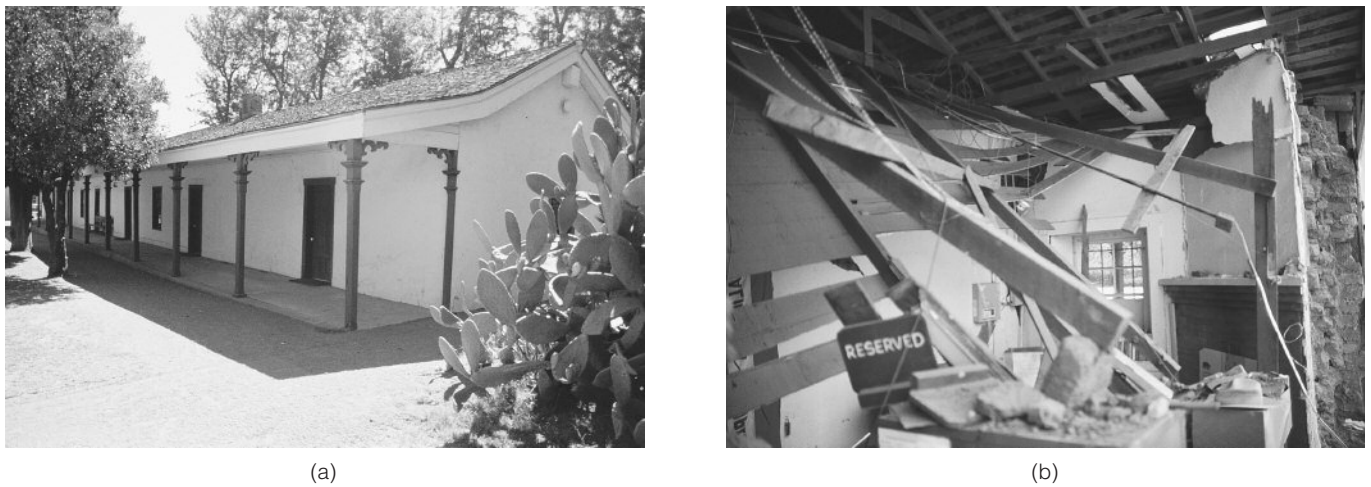
Figure 1.6 De la Ossa Adobe, Encino, Calif.: (a) before 1994 Northridge earthquake, and (b) after 1994 Northridge earthquake.
