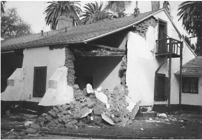
Figure 8.5 Collapsed wall of Ramona's room, Del Valle Adobe.
