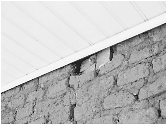
Figure 5.15 Anchorage failure of steel tie-rod; anchor plate has pulled into the wall.
