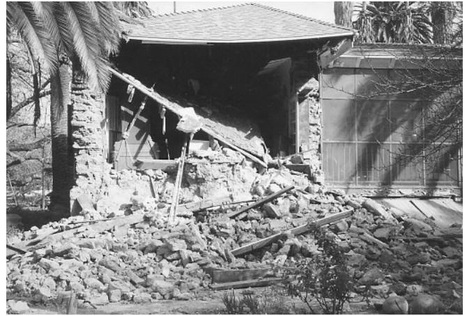
Figure 8.6 Collapsed southwest bedroom wall of Del Valle Adobe.
