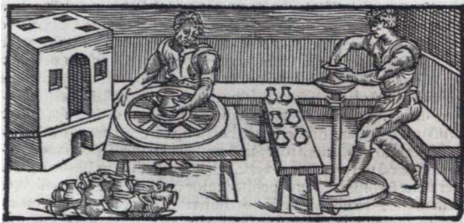
6 Vannoccio Biringuccio. Illustration from chapter 14, book 9, of De la pirotechnia (Venice, 1540). Los Angeles, Getty Research Institute, Special Collections. Two potters use two different types of potter's wheels next to a kiln in their workshop.
