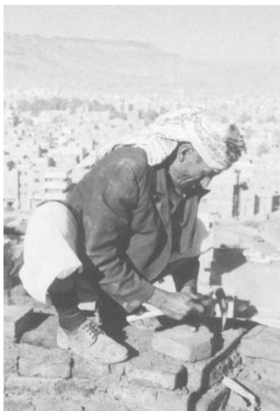
Figure 3 Ahmed al-Maswari, a master mason, perched on top of the walls of the 'Addil Mosque minaret laying bricks (1996). Photo by Trevor Marchand.
