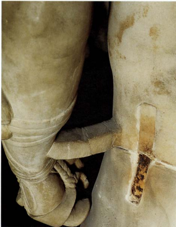
PLATE XIII B | BOURGEOIS Detail of the Pugilist. Roman, second century A.D. Marble, H 1.74 m. Pacetti's restoration, showing marble tassello hiding the iron clamp. Paris, Musée du Louvre MA 68. Photo: A. Chauvet.
