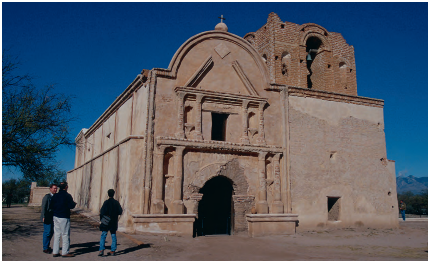
FIGURE 8 Tumacacori, Arizona. Stabilization and early partial reconstruction of the church facade. Photo: Frank Matero
