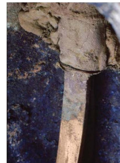
FIGURE 5.10. Upper end of one of the brass bars, wrapped with fabric and attached to the bronze with cement
