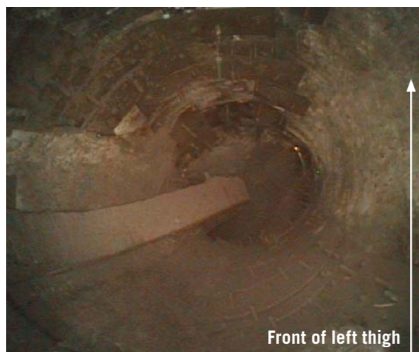
FIGURE 9.24. Videoprobe image looking into the interior of the left thigh, where brass straps and rods repair a long break down both the inseam and outer seam of the leg
